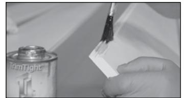
2) Place 1 male panel face up between two female panels along each side. Make sure ends are aligned at top and bottom. Apply PVC Cement to grooves on each side of male panel. Then apply PVC Cement only on that side of each female panel that will be joined with male panel to form a U-shaped column.
