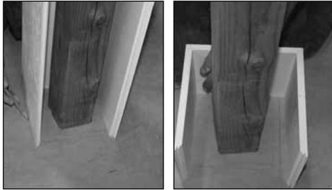
5) Place 3-sided U shaped column around squaring block (as marked) and mark exterior perimeter on floor and ceiling. Remove column and align U-shaped CAP along exterior panel line. Pencil mark interior side.
