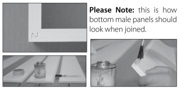
2) Place 1 male panel face up between two female panels along each side. Make sure ends are aligned at top and bottom. Apply PVC Cement to grooves on each side of male panel. Then apply PVC Cement <u>only on that side of each female panel that will be joined with male panel to form a U-shaped column</u>.
