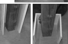
5) Place 3-sided U shaped column around squaring block (as marked) and mark exterior perimeter on floor and ceiling. Remove column and align U-shaped CAP along exterior panel line.Pencil mark interior side.
