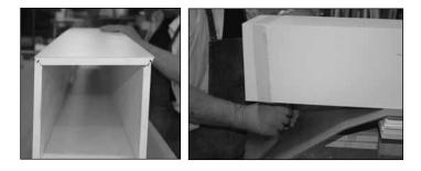
4) Make sure post is level and put squaring blocks into position around post. Measure distance from wall (or other reference
