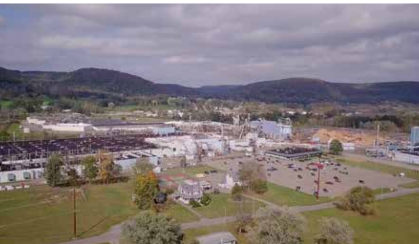
TOWANDA, PA MANUFACTURING FACILITY
