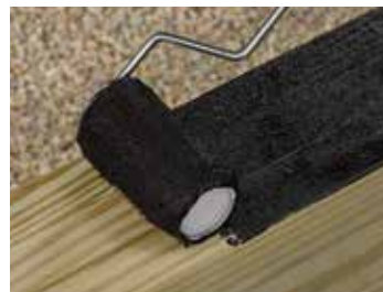
Deck Carrying Beams
