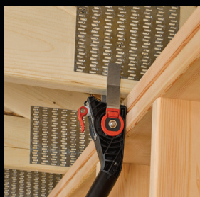
Truss to Top Plate Connection
