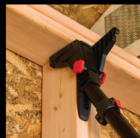
Stud to Top and Bottom Plate Connection
