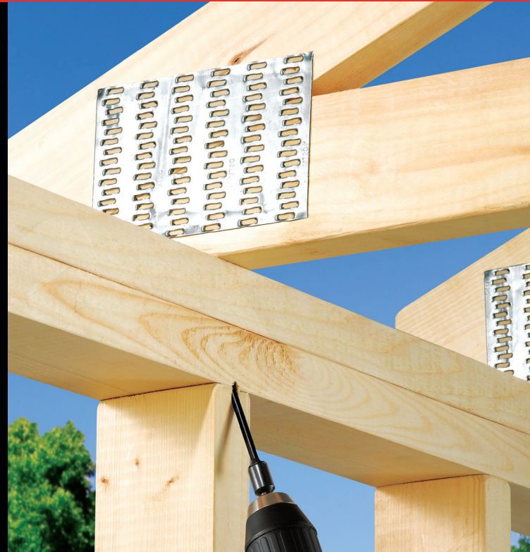
Rafter/Truss to Top Plate
